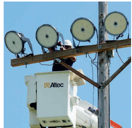
Line Worker Jason Keelin works on getting the new lights properly installed.
