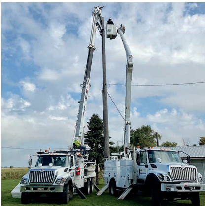
Dakota Energy employees prepare to take down the old stadium lights.
