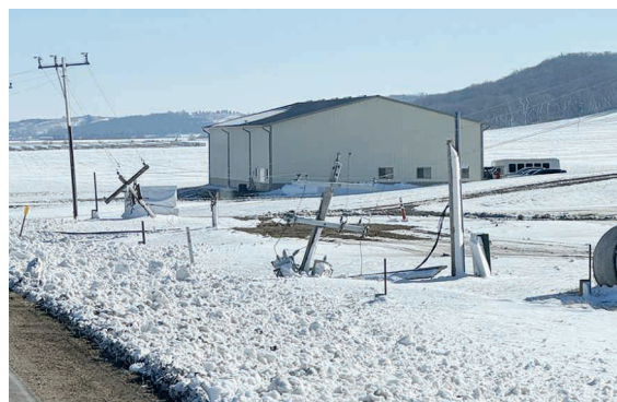
Several three-phase poles snapped off due to the weight of the ice and blowing wind.
