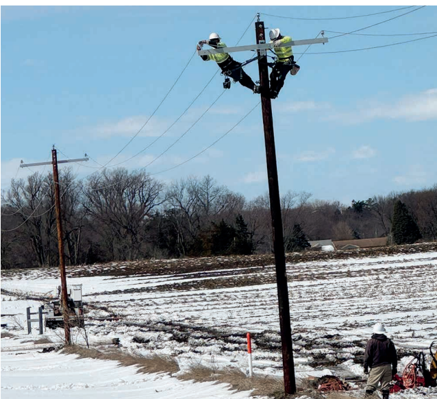
Line workers climbing a three-phase pole to work on crossarm.
