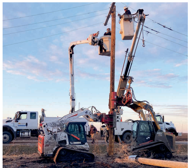
Line workers setting a three-phase pole.
