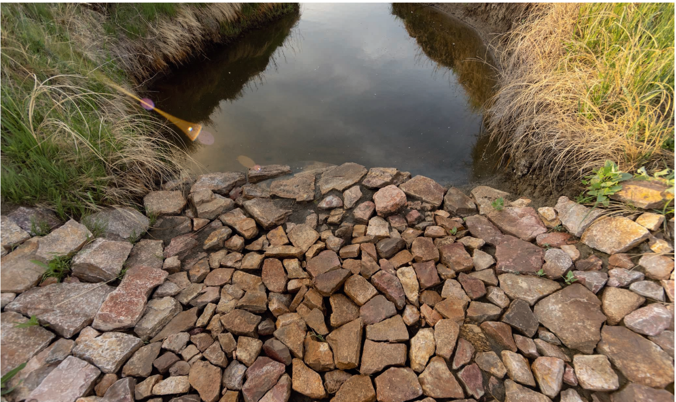
A rock structure installed to help prevent headcuts from eroding upstream reaches. Photo Credit: Joe Dickie, Generation Photography, Inc.
